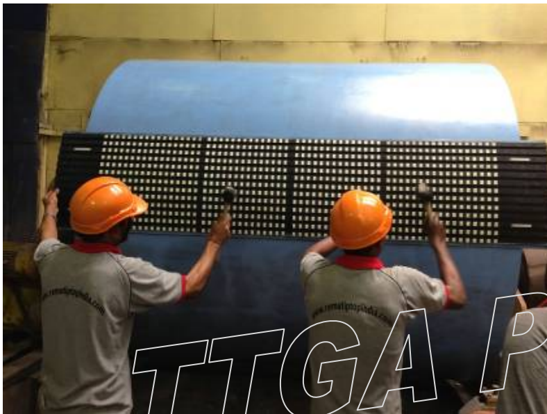
Bonding of Remagrip CKX HD
